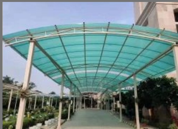
Polycarbonate Sheet Roofing Installation Service
