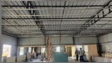
PVC Sheet Roofing Installation Service
