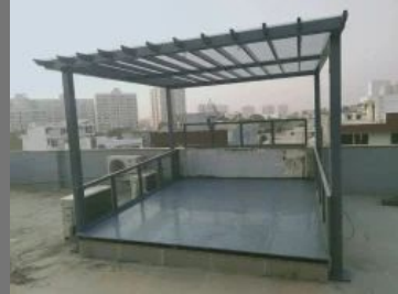
FRP Sheet Roofing Installation Service
